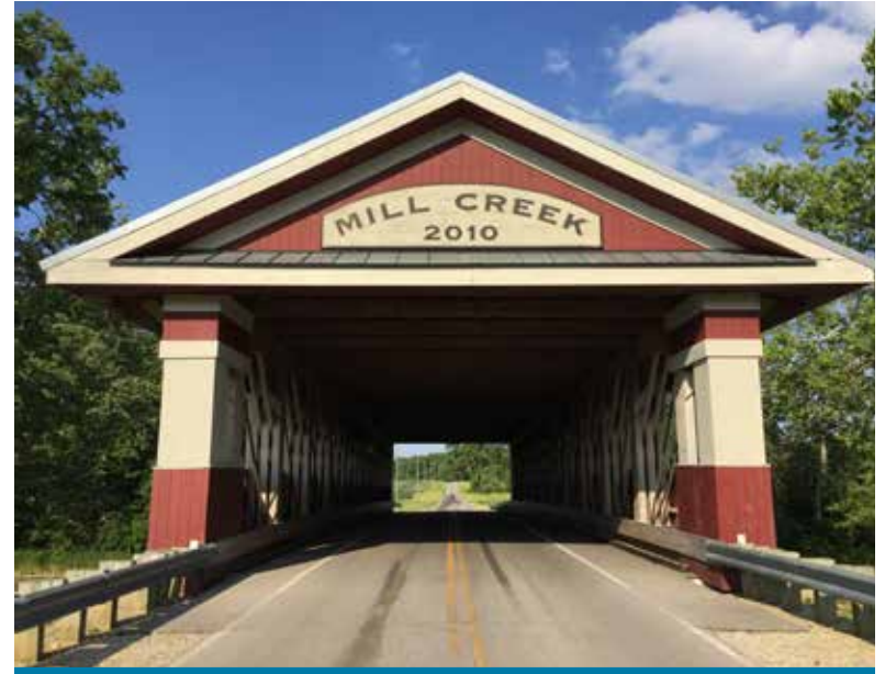
The 2025 update to the Millcreek Township Comprehensive Plan re-establishes the community's vision and will help to support community decisions for years to come. The Township intends to remain a predominately rural community, that maintains its agricultural heritage and independence.
